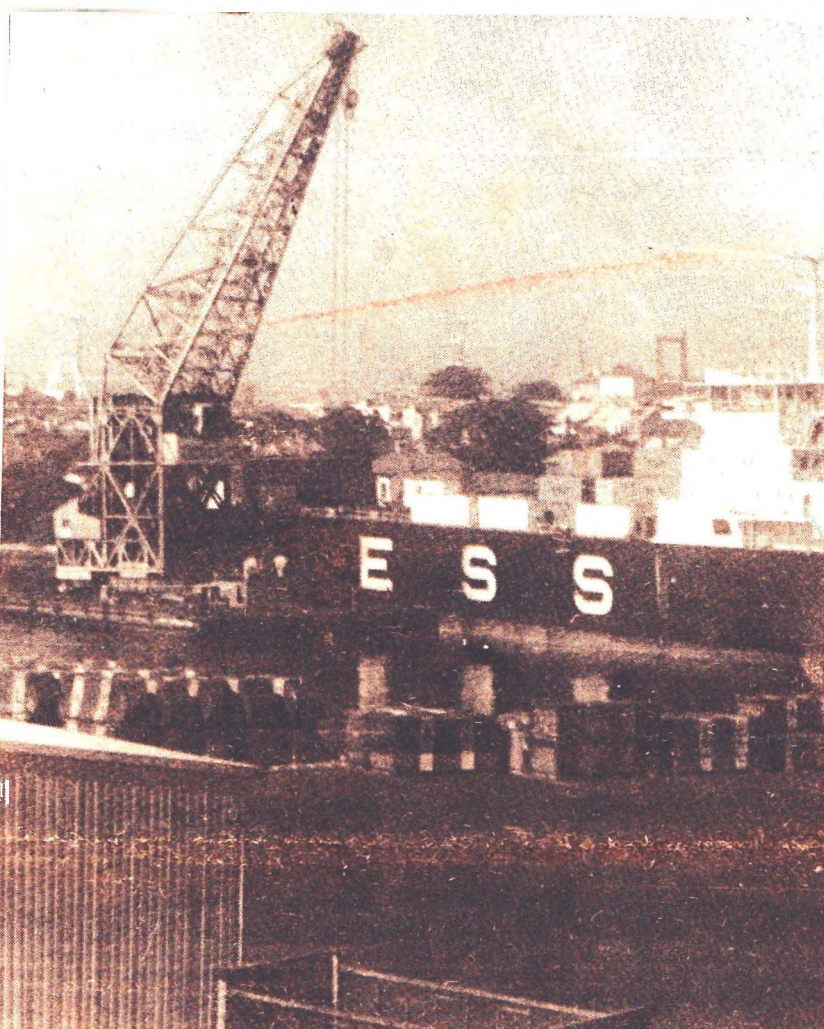
SCOOP! The Link shows the floating Titan crane being used to unload heavy equipment from the Matthew Flinders onto a barge at the ANL terminal at Mort Bay.
