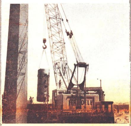
A little piece of old Balmain departs! This picture shows a crane fishing out one of the old boilers of Balmain Hospital which has ended its useful life. It had to be taken out through the roof of the building it occupied.
